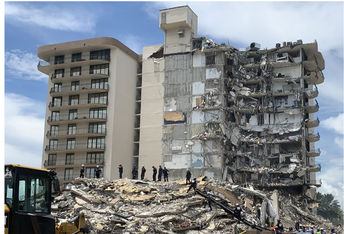
The site of the Champlain Towers South partial collapse in Surfside, Florida.
