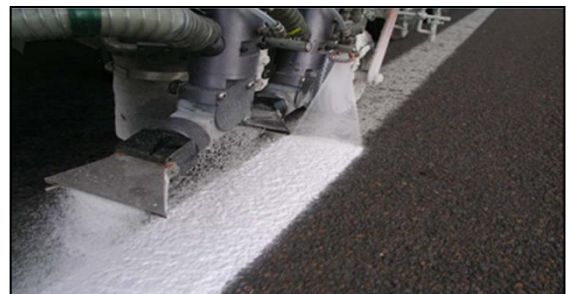
Figure 3: Example of recycled glass used in highway paint
